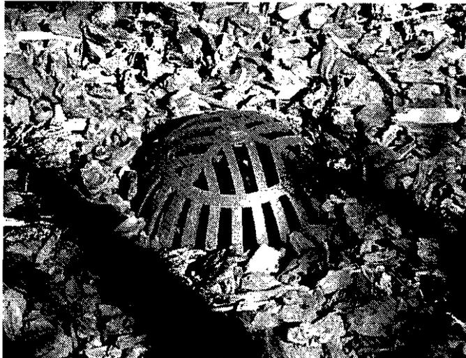
Remove debris from area drains
