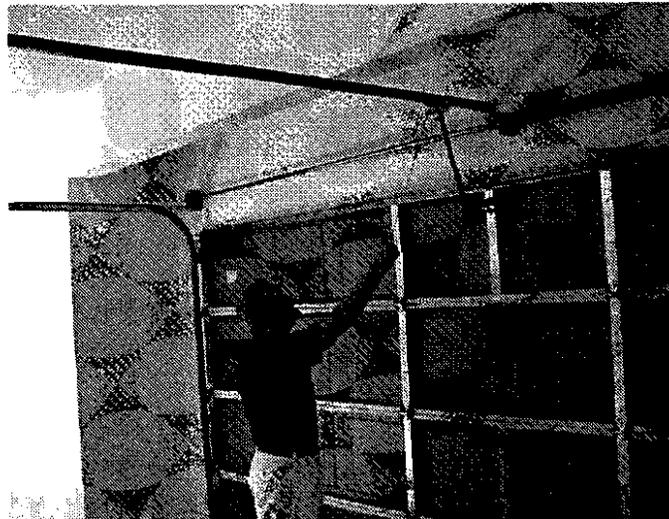
Disconnect the door and manually check balance; it should open and close with minimal effort
